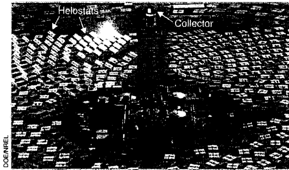
Figure 9. large-scale, central receiver, solar thermal installation: 10 MW Solar Two installation in the Mojave Desert, California.
