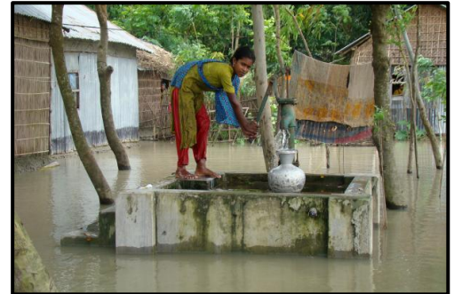
Water pump built on a raised plinth
