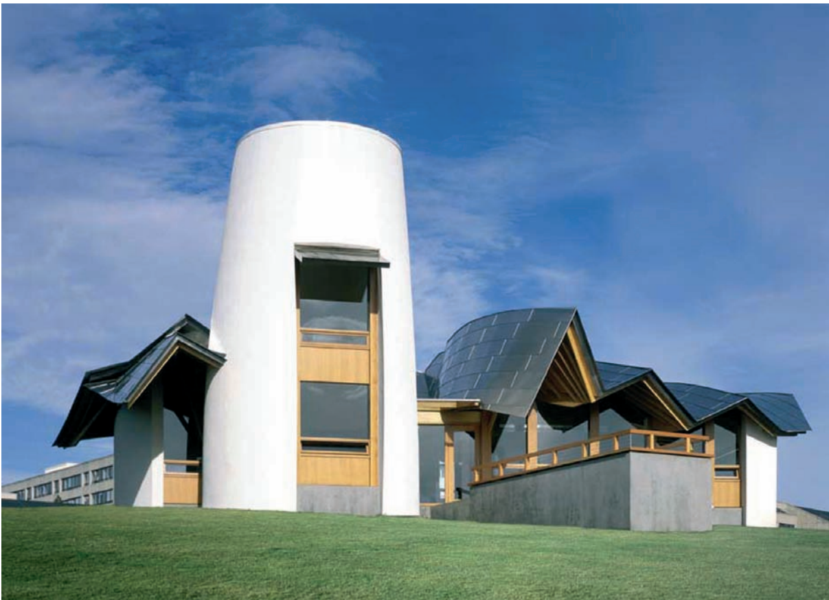
Maggie's Centre , Dundee, designed by Frank Gehry (2004) Materials: stainless steel roof, reinforced concrete and wood.
