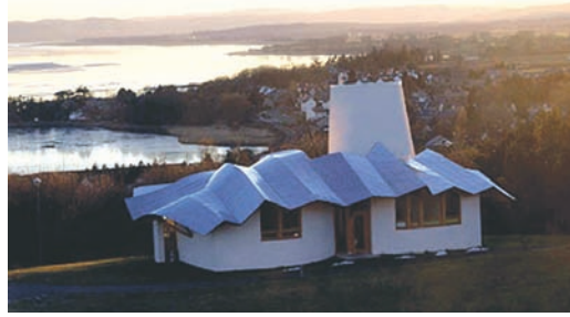
View of rear of Centre and surrounding area
