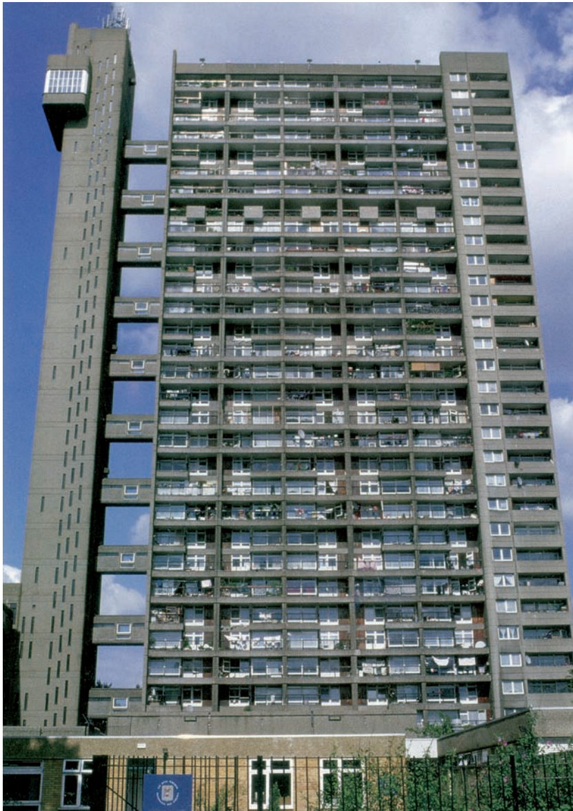
Trellick Tower , London, designed by Erno Goldfinger (1972) Materials: reinforced concrete and glass.
