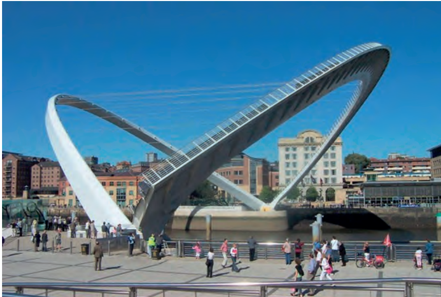
Millennium Bridge , Gateshead, (2001) designed by architects, Wilkinson Eyre and structural engineers, Gifford
