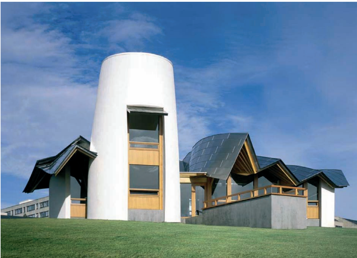
Maggie's Centre , Dundee, designed by Frank Gehry (2004) Materials: stainless steel roof, reinforced concrete and wood.
