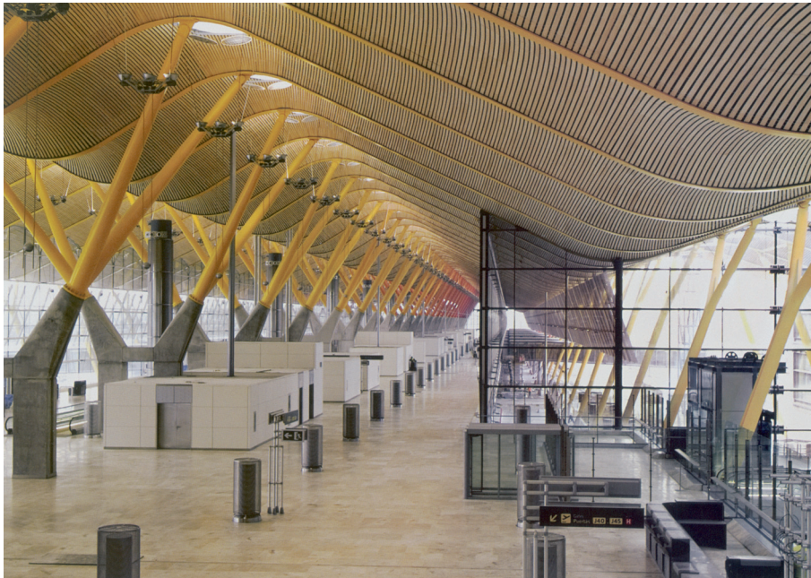
Barajas Airport Terminal , Madrid, designed by Richard Rodgers Partnership (2006).
