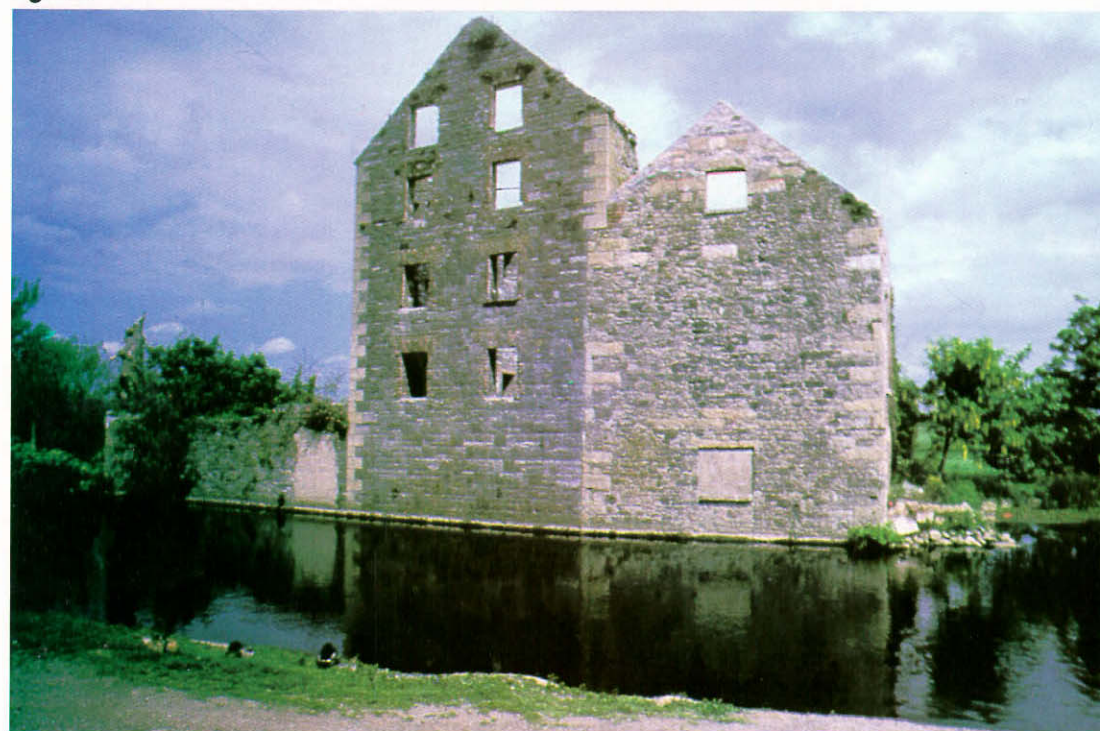
Canal Side Building
