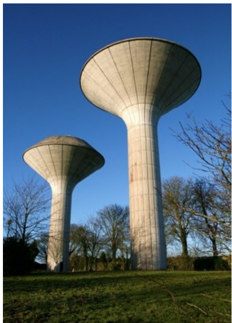
Typical Water Towers
