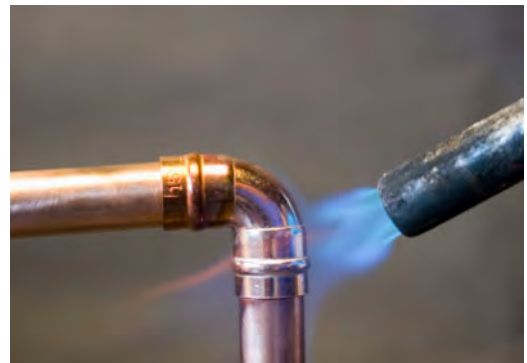
Plumbing a solder fitting
