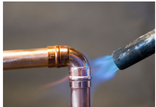
Plumbing a solder fitting
