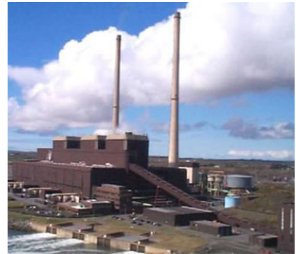
Moneypoint Power station
