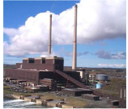
Moneypoint Power station
