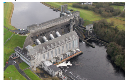
Hydro-Electric Power Station
