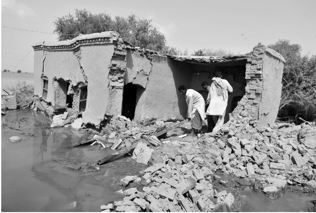
Earthquake Damage in Pakistan (2010)
