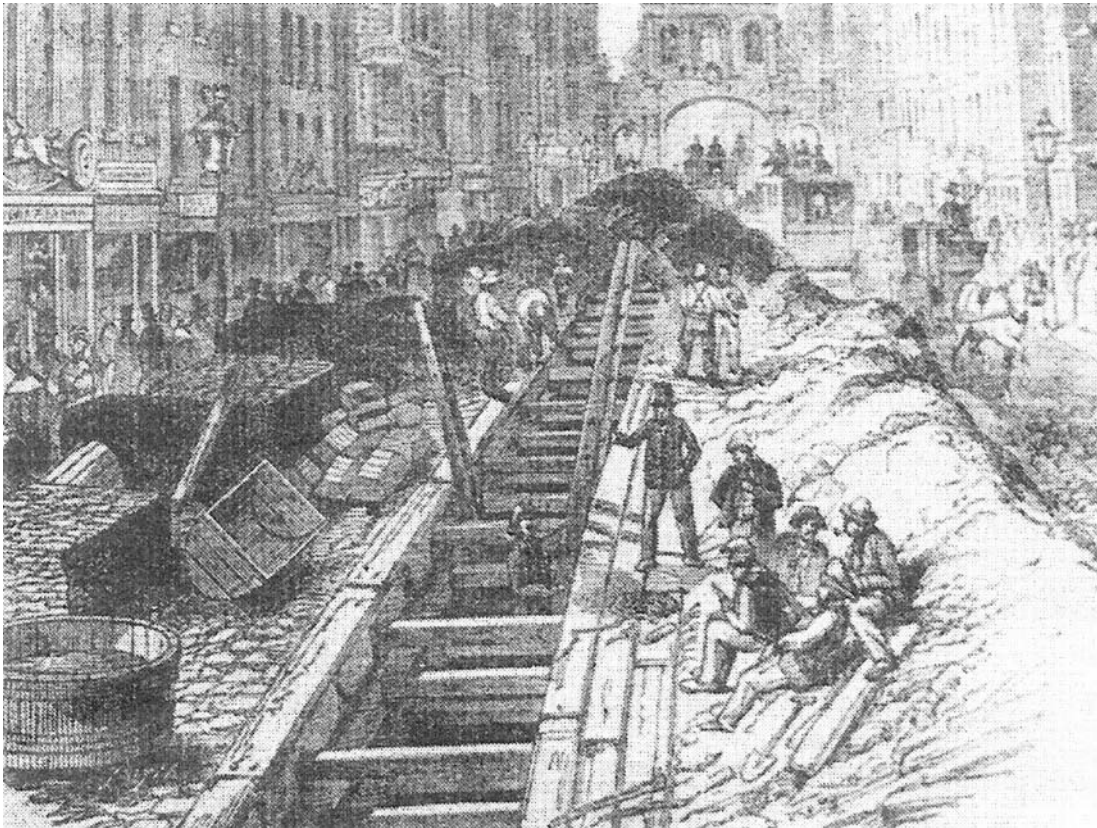
Building a sewer in London in 1844.
