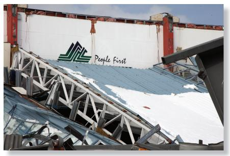
Figure 6: Collapsed roof of Stadium Southland in New Zealand
