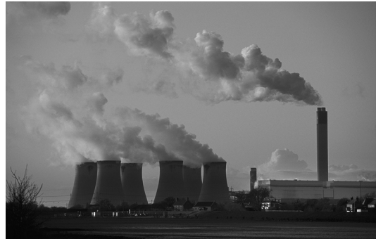
Coal-fired Power Station
