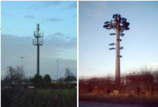
Masts like this one are Some are disguised used to 'boost' signals to mobile phones within tree!). a radius of about 25 -30 miles.
