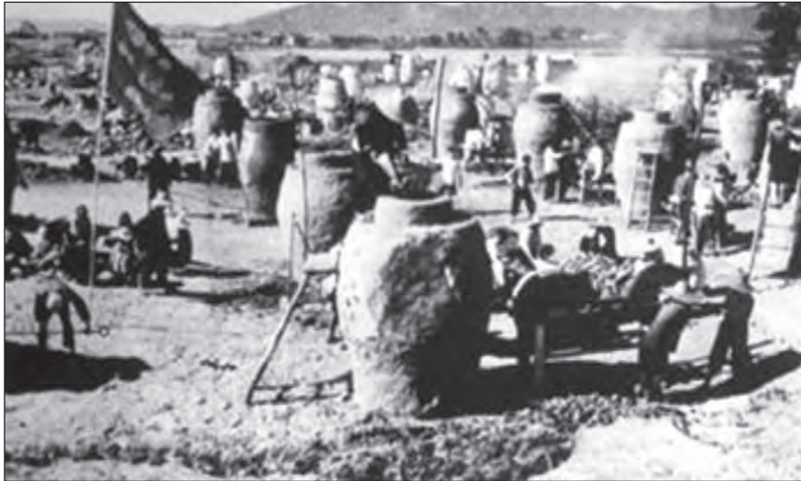
[The photograph shows backyard steel furnaces in the late 1950s]
