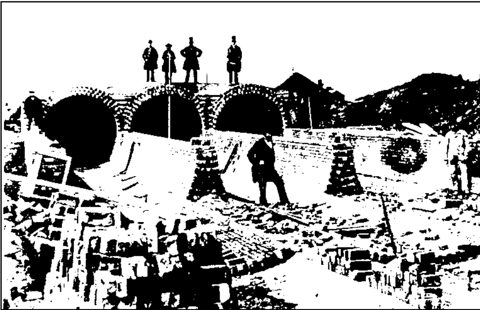
A photograph of sewers being built in London in 1862.
