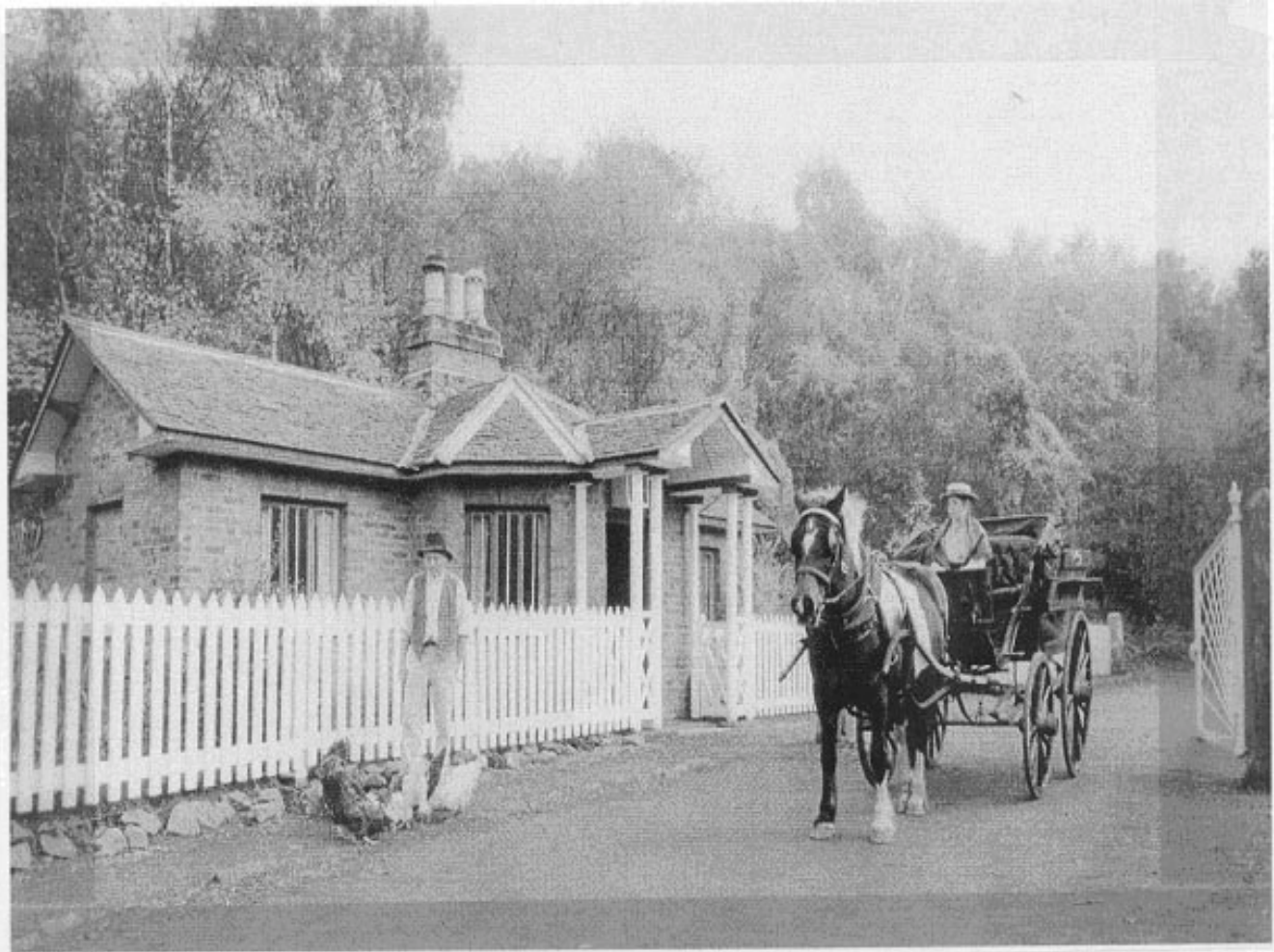
SOURCE J: A reconstruction of Telford’s Shelton tollhouse at the Blists Hill Museum in the 1970’s
