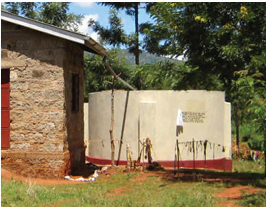
Fig. 7b Rain water storage tank
