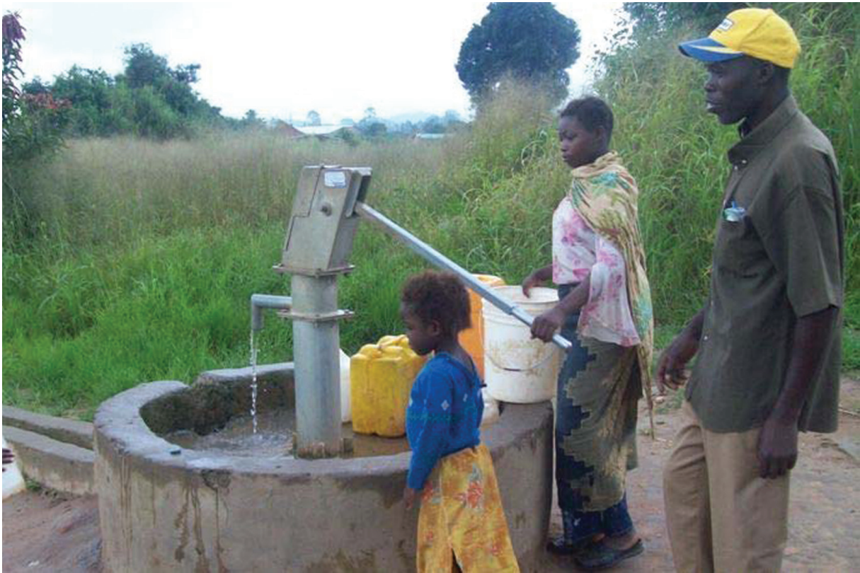
Fig. 7a Groundwater supply water pump
