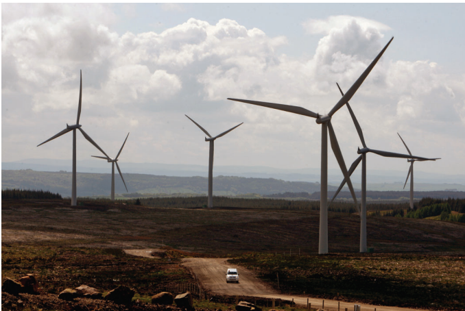
Onshore wind farm at Eaglesham, Scotland
