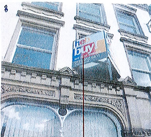
For let and sell Signs on empty buildings.
