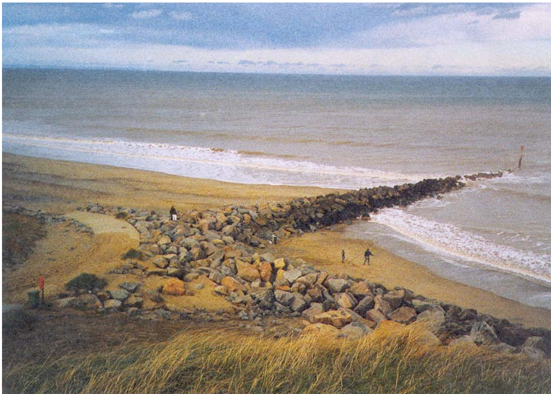
Photograph D – Rock groyne at Mappleton
