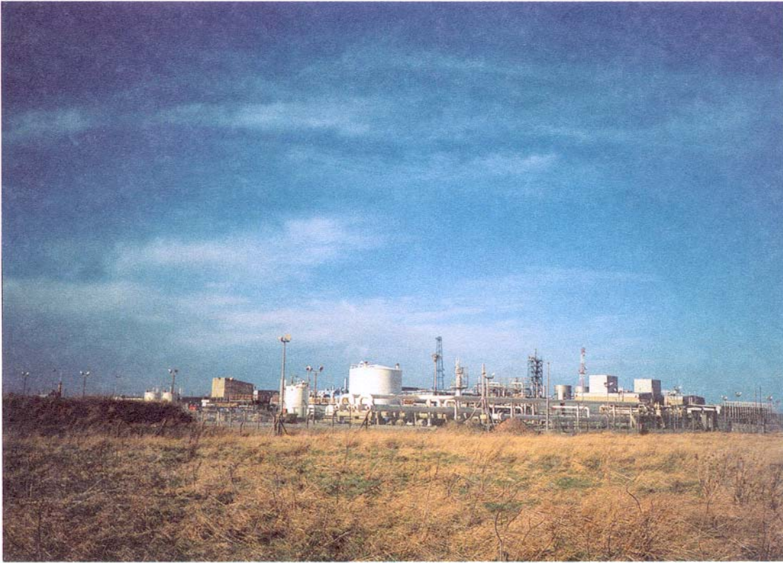
Photograph H – Easington Gas Terminal
