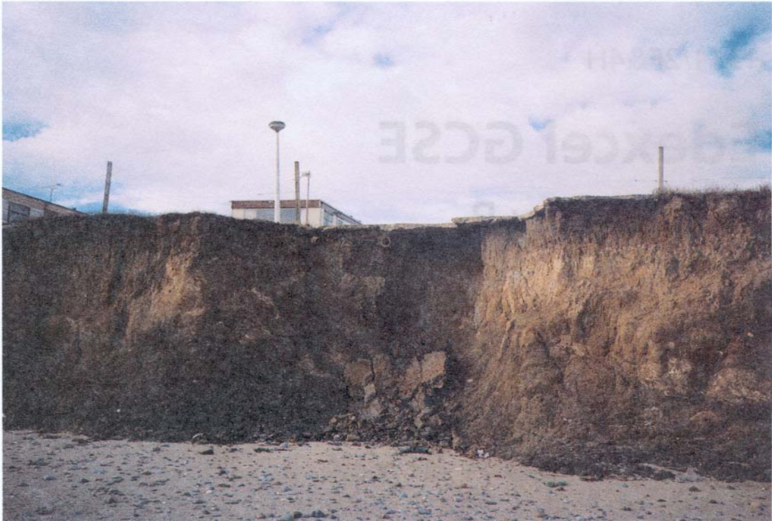
Photograph A – Easington cliff and beach
