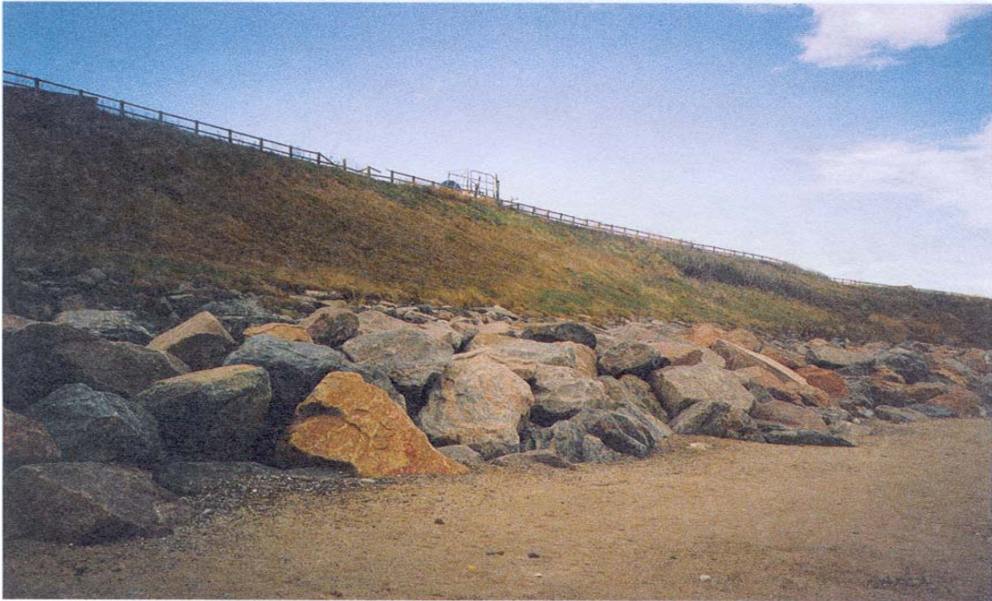
Photograph C – Rock revetment and graded cliffs at Mappleton
