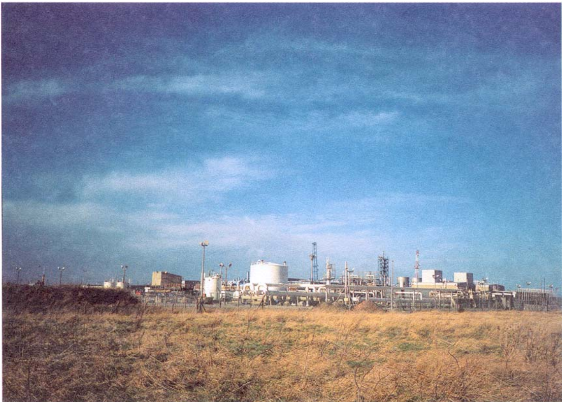
Photograph H – Easington Gas Terminal
