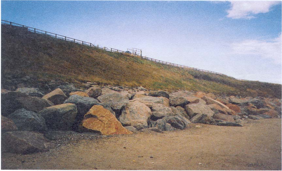
Photograph C – Rock revetment and graded cliffs at Mappleton
