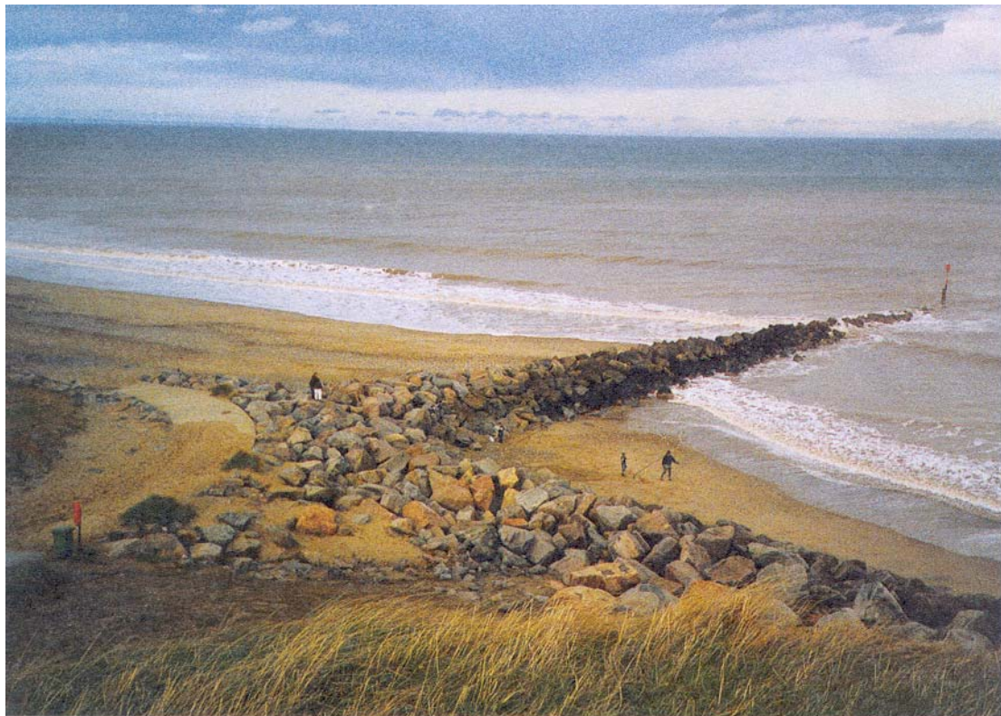
Photograph D – Rock groyne at Mappleton
