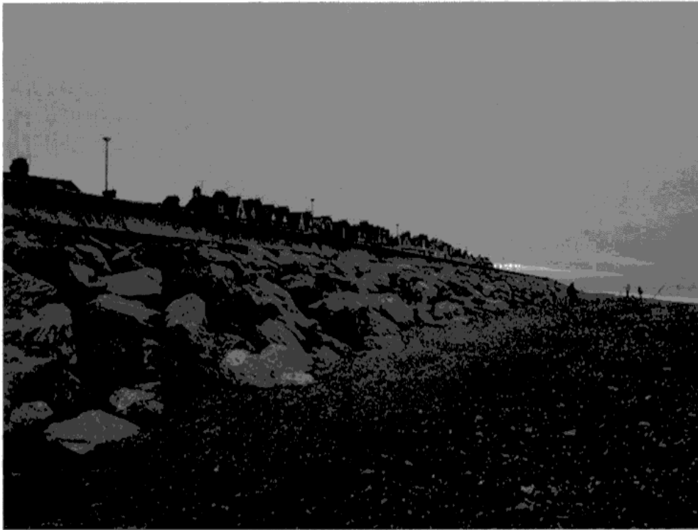
Figure 5 – Photograph of Coastal Defences
