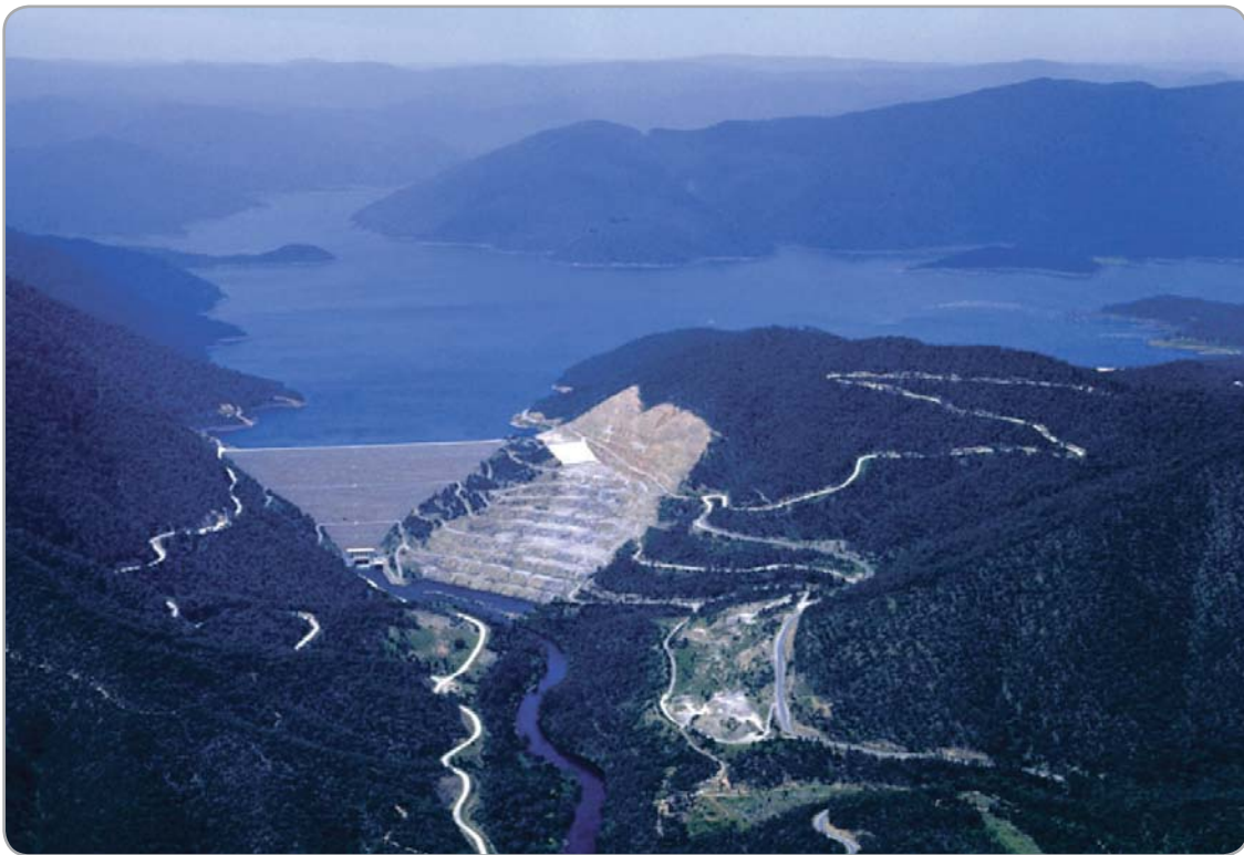
Figure 15 The Dartmouth Dam and reservoir, part of the Snowy Mountains Scheme
