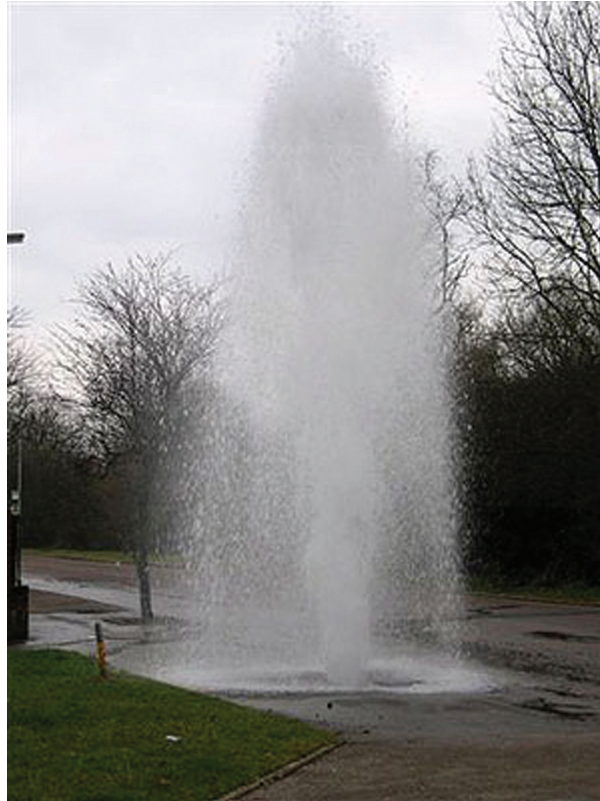
Photograph E. Water loss from a burst water pipe in London.
