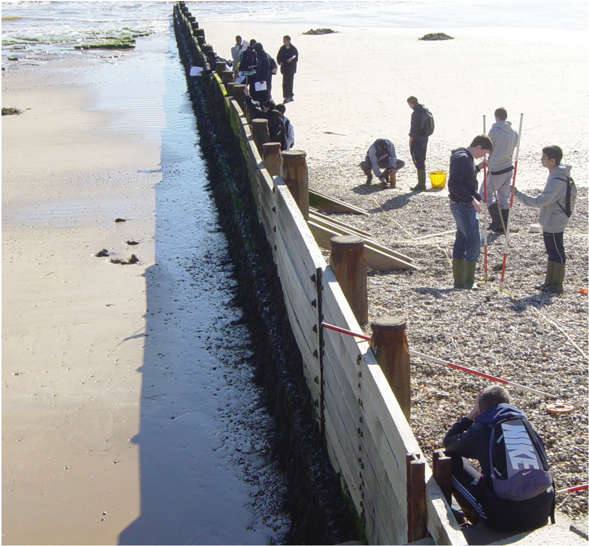
Photograph A. Students studying groynes, an example of hard engineering at the coast.
