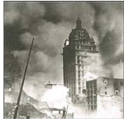
Fire engulfs the Call Building
