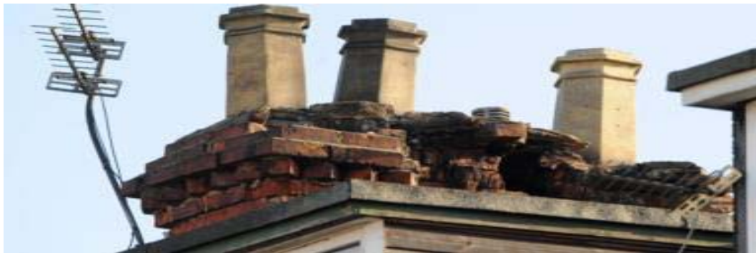
A chimney stack on a house in Goole, East Yorkshire, that was damaged by the earthquake
