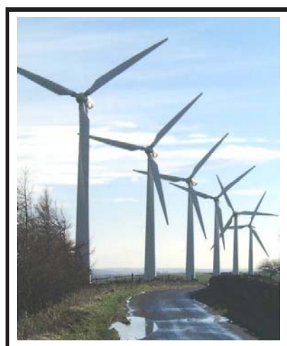
STARTING POINT: Wind Farm
