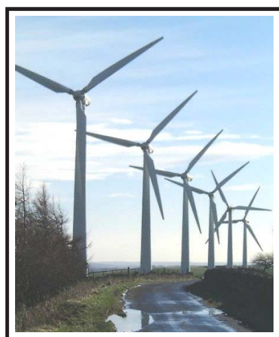
STARTING POINT: Wind Farm
