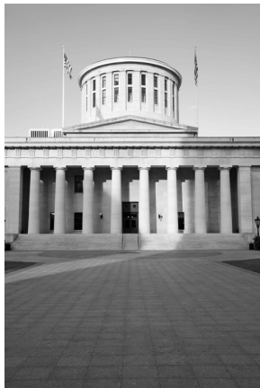
This building is made from limestone. Limestone is calcium carbonate. Limestone is a soft and crumbly rock.
