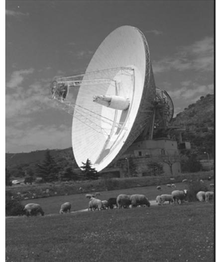
Radio signals weaken as they travel from a deep space probe across the great distance to Earth. Receiving antennas on Earth must have greater reflecting surface to pick up the weak signals. The signals are so weak it is important to use digital signals.
