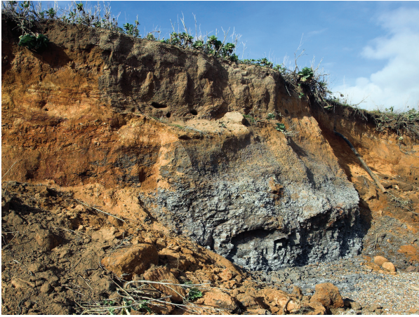
Photo 1 Cliff regrading high maintenance and high cost.
