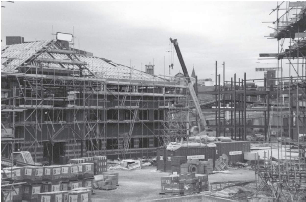
Three-storey office development project
