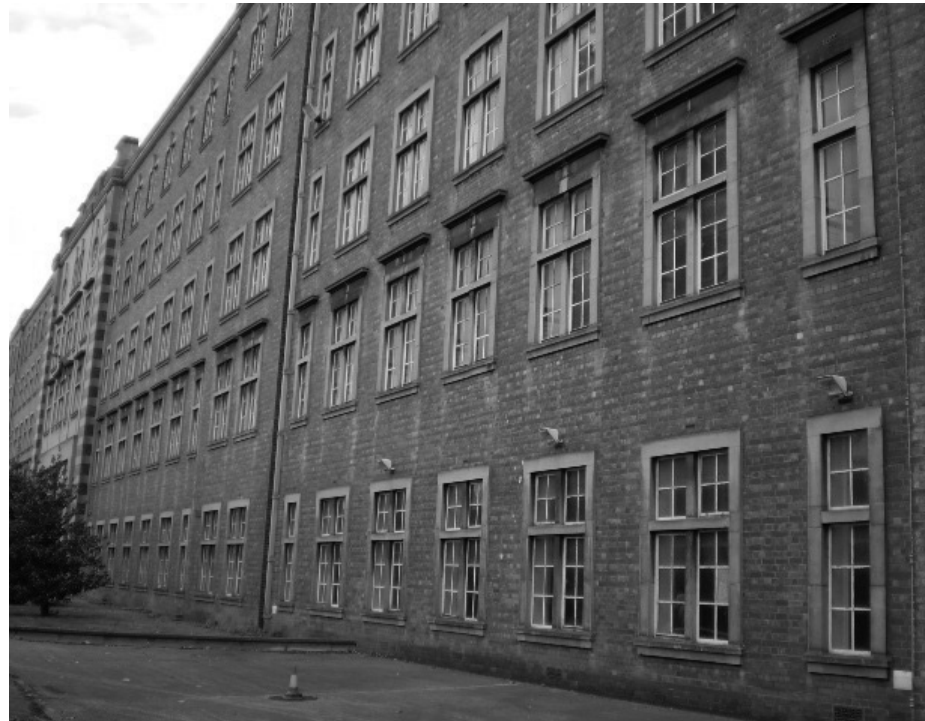
Existing five storey factory building
