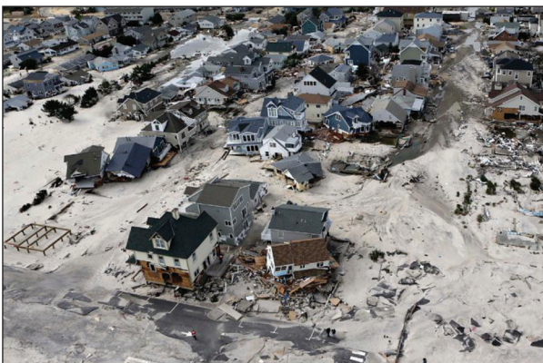
Seaside Heights was damaged by coastal flooding in 2012
