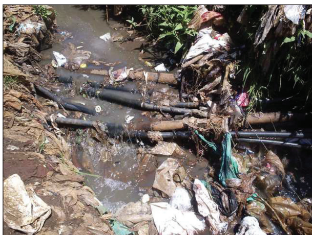
Old water pipes crossing a sewage trench
