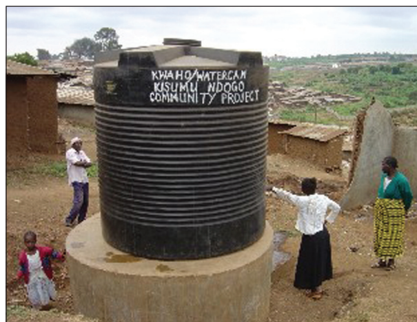
New, safe water storage tank
