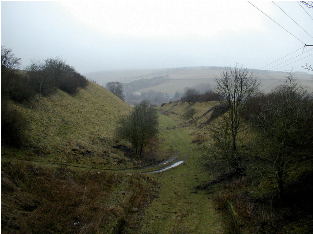
PHOTOGRAPH D The route of the Waverley railway project route at Stow, showing an overgrown cutting of the original line
