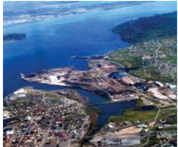
Sydney steelworks site being cleared, 2004
