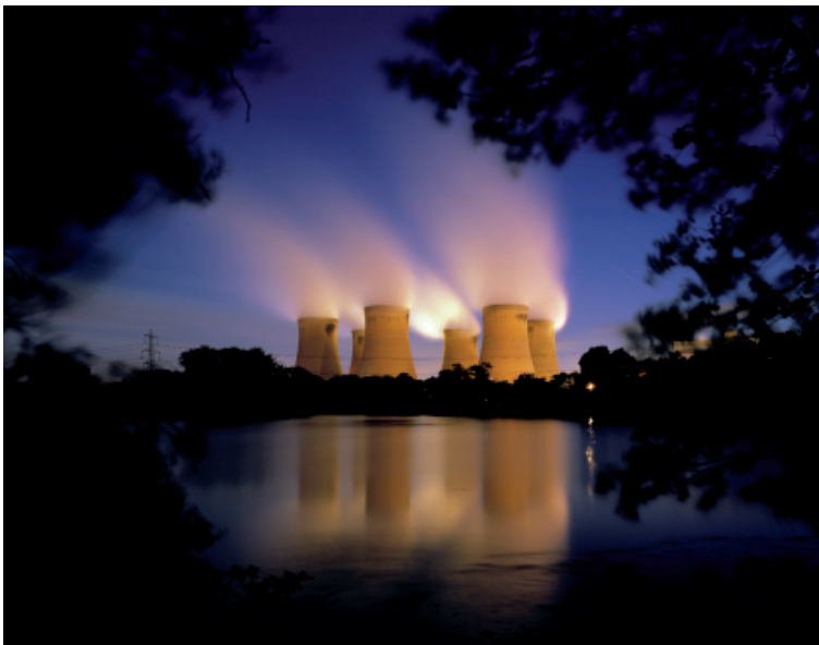
Drax, the largest power station in the UK providing 7% of Britain's power
