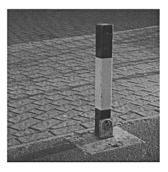
Height of bollard =  $1000 \, \text{mm}$ Cross-section of bollard =  $80 \, \text{mm} \times 80 \, \text{mm}$ Mass of bollard =  $10 \, \text{kg}$
