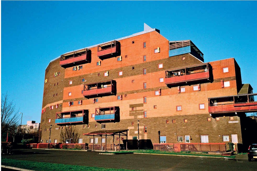
Byker Wall by Ralph Erskine 1987 Newcastle upon Tyne
