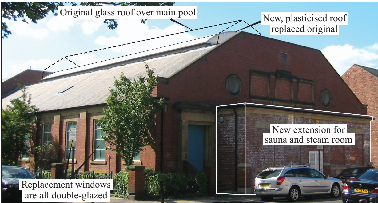
Figure 2 – Jesmond Pool (view from North), September 2006
