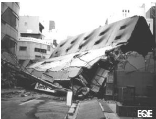
Blocked street in central Kobe
