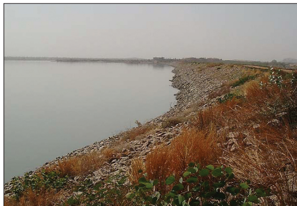
A national option: building the Kafin Zaki Dam
