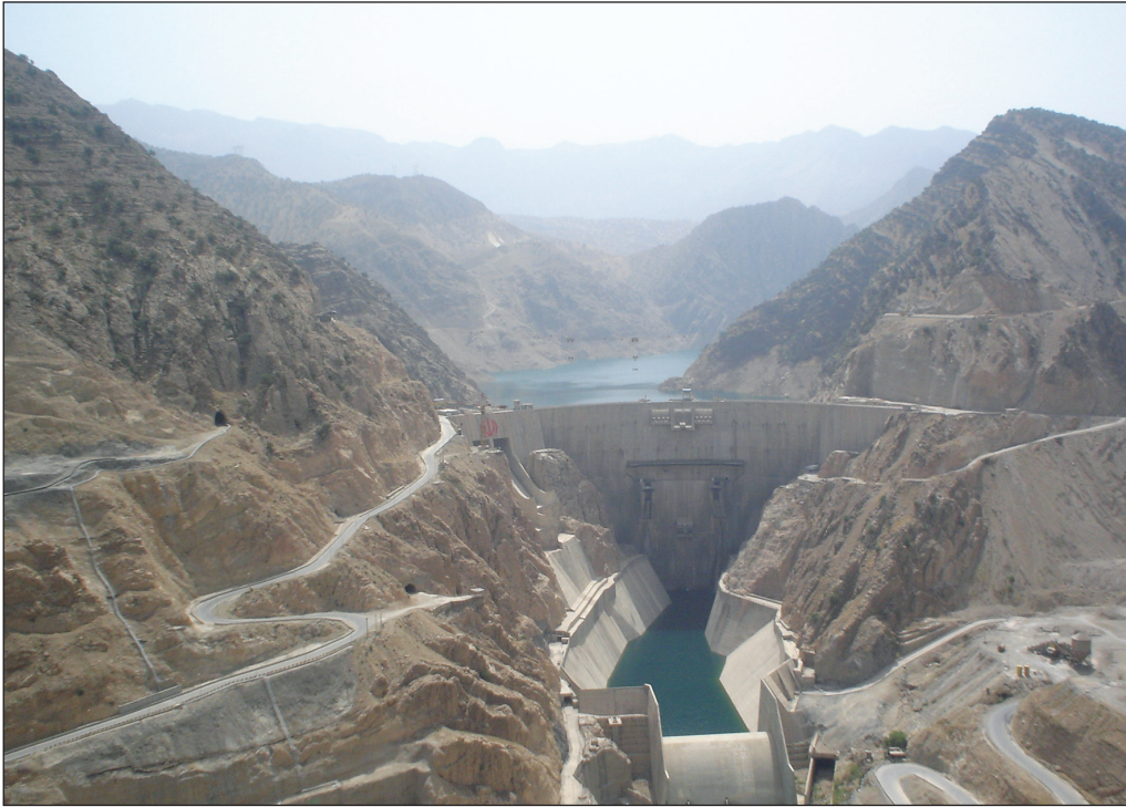
Figure 24: The Karun III dam in Iran
