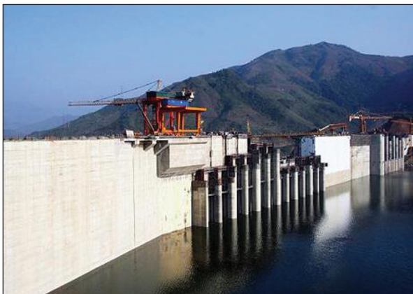
HEP station under construction in Vietnam
