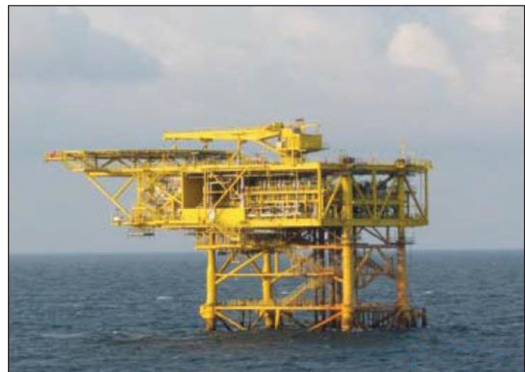
Gas platform off the coast of Vietnam
